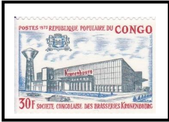
The Kronenbourg plant in the Congo.
